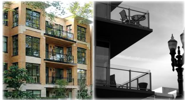
Balconies should be recessed/integrated into the facade of low-rise buildings. Projecting balconies should use clear glazing.
