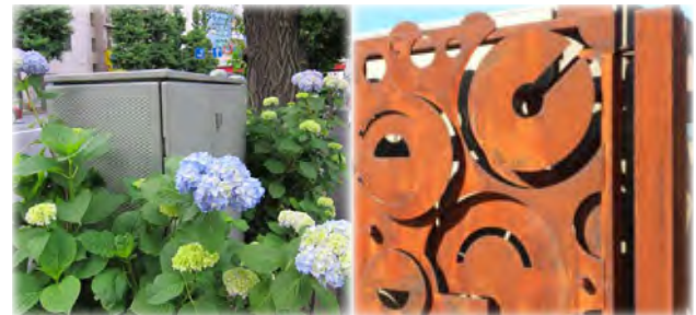
Surface utility equipment can be screened with dense landscaping or decorative casings.
