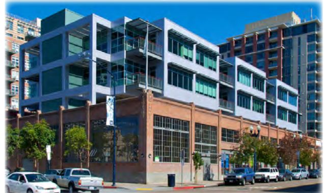
Additions or significant alterations to historic building should be visually distinguishable from the original structure.
