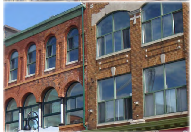
Use mouldings, brickwork, sills and other details to add depth and character to windows.
