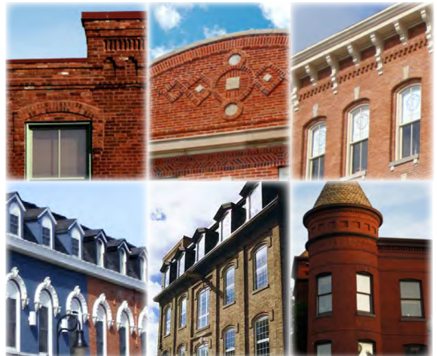
Create distinctive and varied rooflines which also serve to screen views of any rooftop mechanical equipment.
