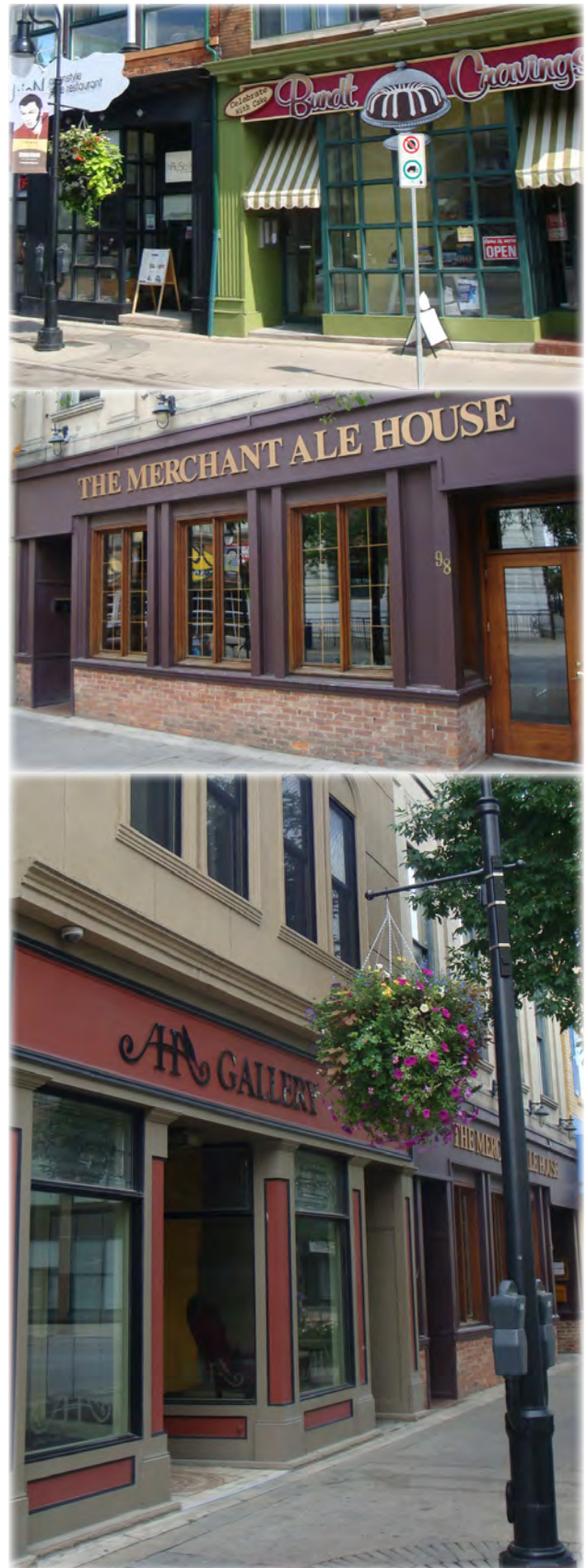
Example Downtown storefronts with large clear display windows, recessed entrances, cornice, sign band, and base panels.
