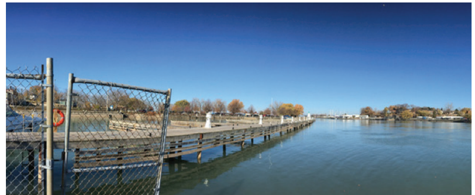
2h Panoramic view from the end of Harbour Walk, boat mooring, buildings on Lakeport Road, Lakeside Park, Harbour entrance and lighthouses in distance. (Catherine Nasmith)
