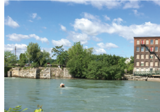
4a Part view of Maple Leaf Rubber and the stone walls of the former Welland Canal. (Catherine Nasmith)
