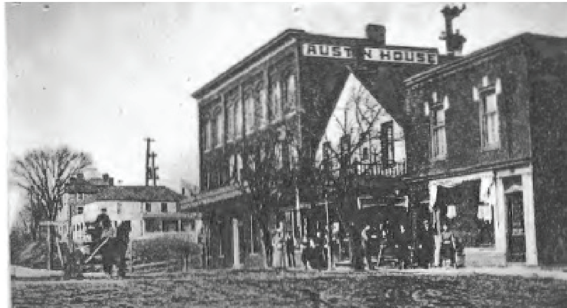
Late 19th century view of Lock Street, note muddy character of street and building, now missing next to the former Stanton Grocery and Post Office Building
