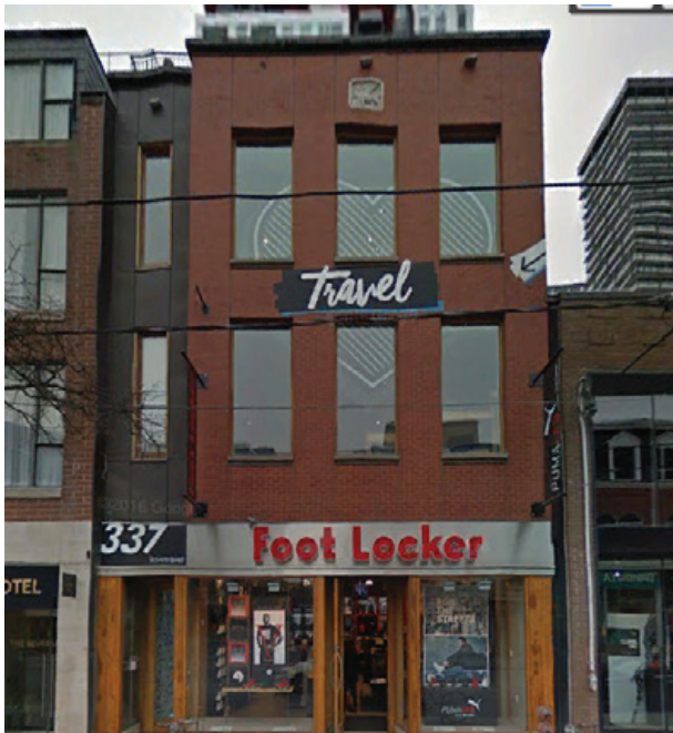
Contemporary yet compatible and respectful infill commercial building from Queen St W in Toronto (Google Earth)
