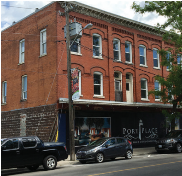
16 Lock Street, the former Lakeside Hotel retains some interior features which may warrant designation of the property under Part IV of the Ontario Heritage Act (Catherine Nasmith)
