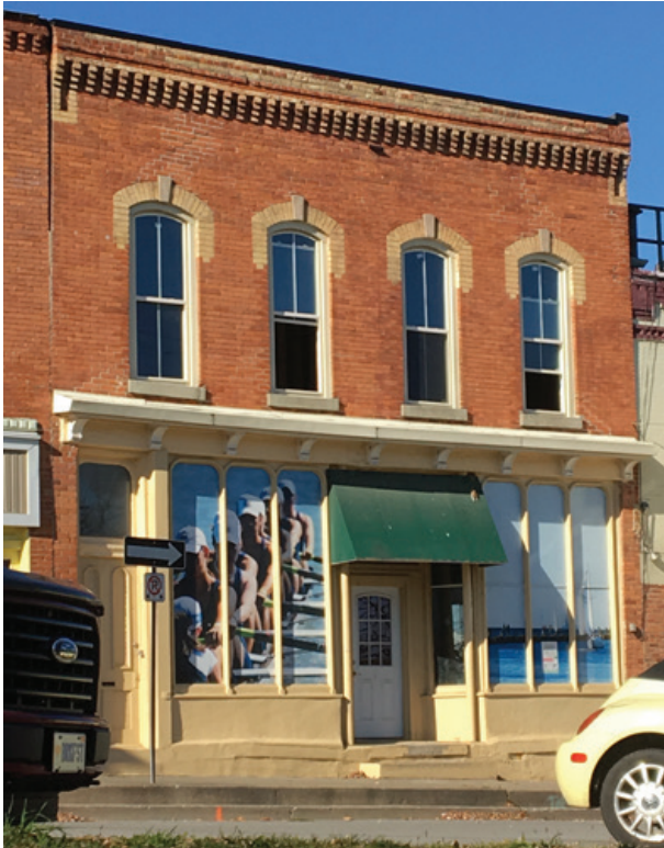
Commercial Building (former Dwyer's Grocery) in Italianate style built on the former Front Street, 18a Lakeport Road, has a well preserved shop front typical of the style (Catherine Nasmith)
