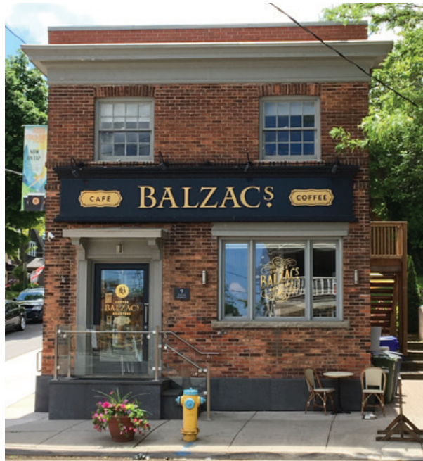
Former Stirling Bank building, 1907, simple handsome brick commercial building, with heavy wood cornice
