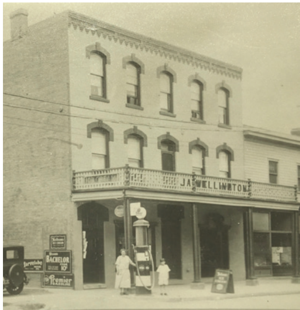
Lock Street c. 1920, Wellington Hotel: verandah, and sidewalk directly in front of hotel, but basic footpath to the east
