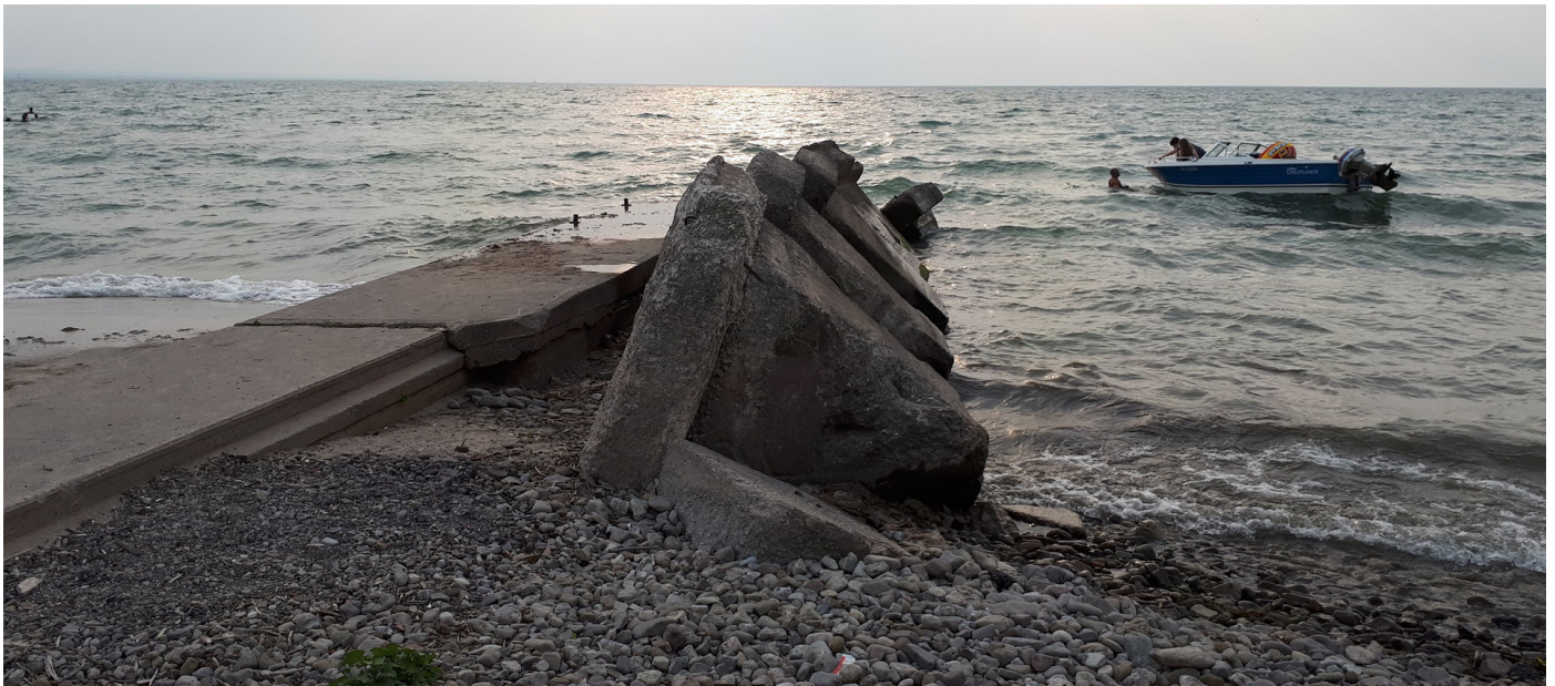
Boat Launch showing detail of break wall
