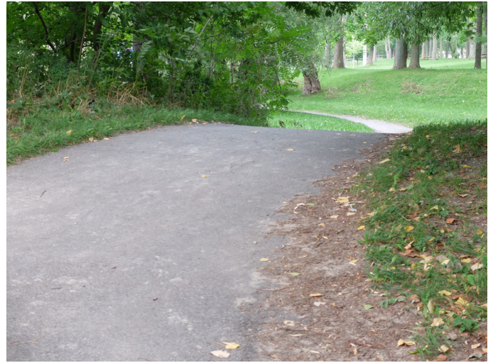
Trail near Arthur Street is steep at this location
