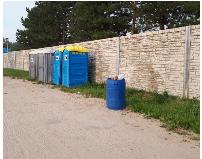
Existing condition at back of parking area.
